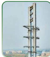
220kV Multi Circuit Tension/ Dead End Dual Pole
