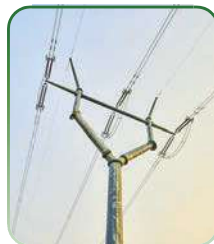
400kV S/C "Tension/Dead End" Y-Pole
