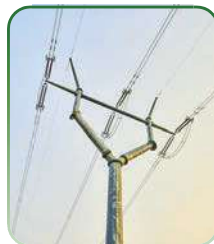
400kV S/C "Tension/Dead End" Y-Pole
