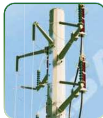
220kV Double Circuit Cable Termination Pole
