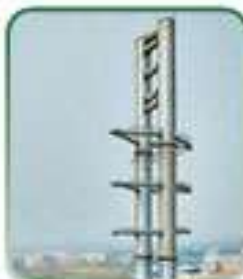
220kV Multi Circuit Tension/ Dead End Dual Pole MSETCL (Maharashtra State Electricity Transmission Company Ltd.), Mumbai
