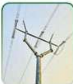
400kV S/C Tension/Dead End Y-Pole PCIL (Power Grid Corporation of India Ltd.), Lucknow
