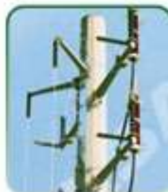
220kV Double Circuit Cable Termination Pole MSETCL (Maharashtra State Electricity Transmission Company Ltd.), Mumbai
