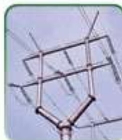
400kV Double Circuit Tension Dead End Y-Pole MSETCL (Maharashtra State Electricity Transmission Company Ltd.), Mumbai
